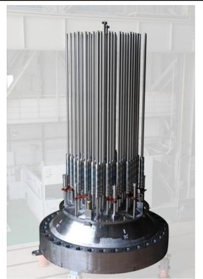
An illustration of a nuclear reactor head, similar to what will be installed at the Davis-Besse plant.
